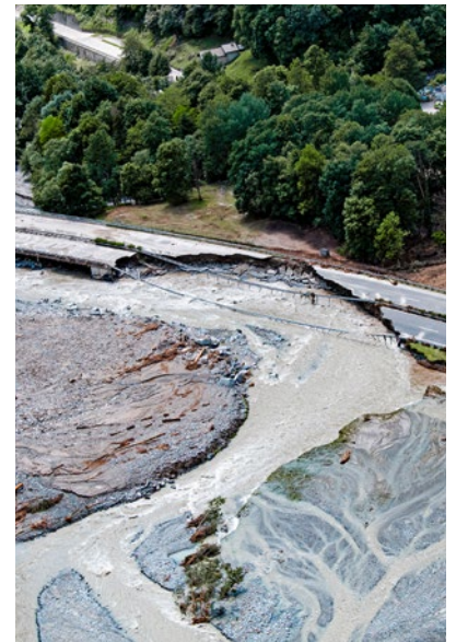
Right: Heavy rainfall in southern Switzerland caused widespread destruction in the summer of 2024. The picture shows a section of the A13 near Lostallo in the Miso Valley that was washed away.
