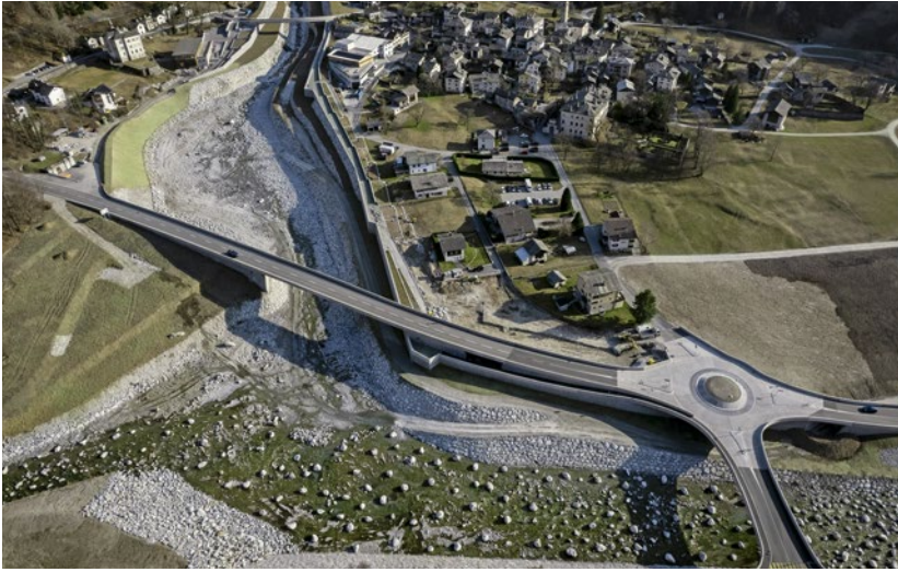
Top: In Bondo (Grisons), authorities have invested 50 million Swiss francs in protective structures, including a dam and a catch basin. In 2017, the village was razed by a mudslide.
