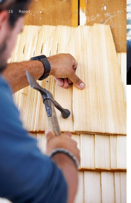
Have the shingles been laid properly? Tristan Ropraz checks the surface he has just laid, which will keep out the wind and weather for 35-40 years.
